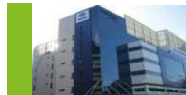
Tata Communications Exchange
