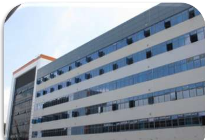
Completed 6-storey extension wing
