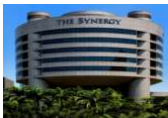
Business Park Buildings
